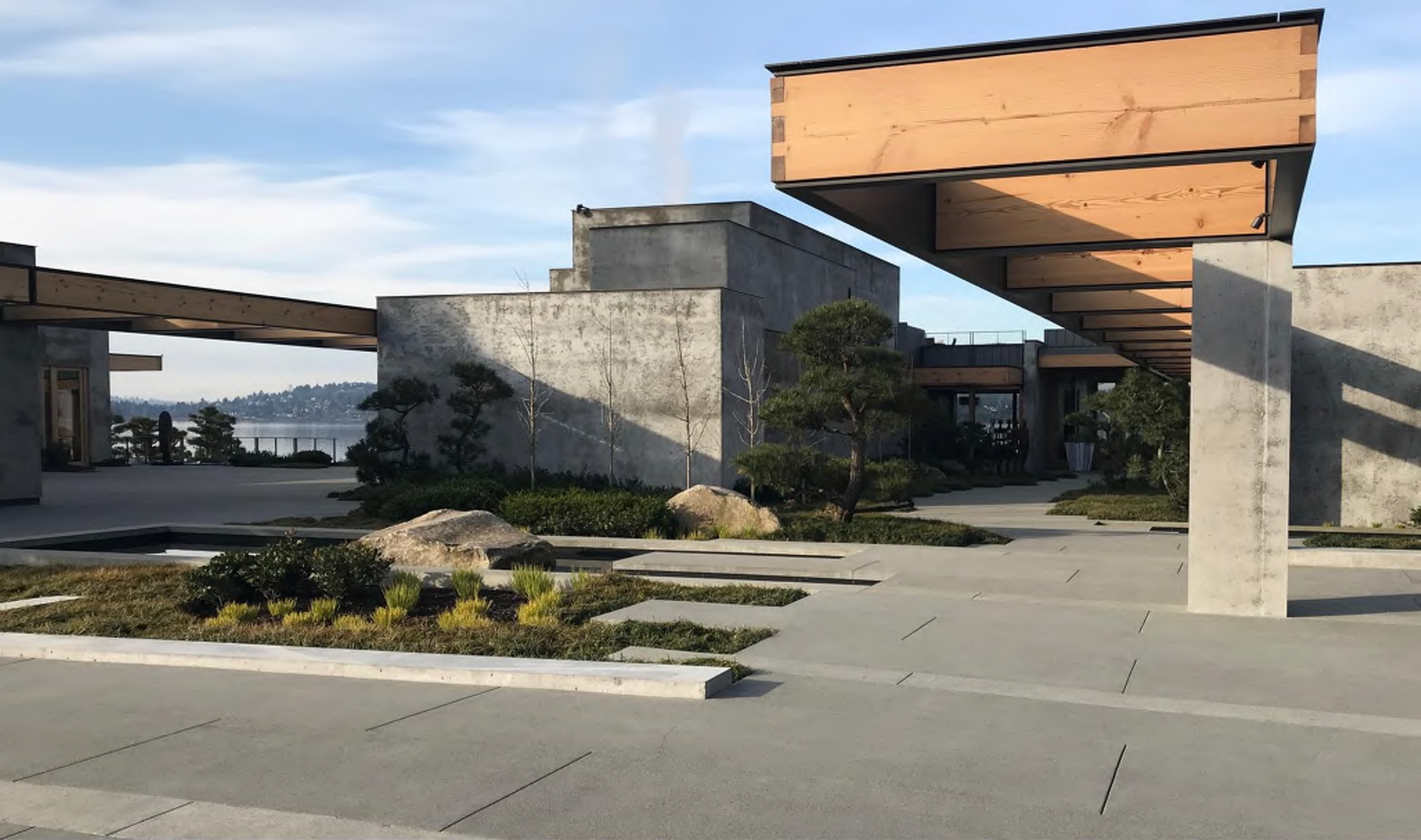
Architect Susan Desko AIA | PROCTOR LANDING | Mercer Island, WA | Project Type: Renovation
