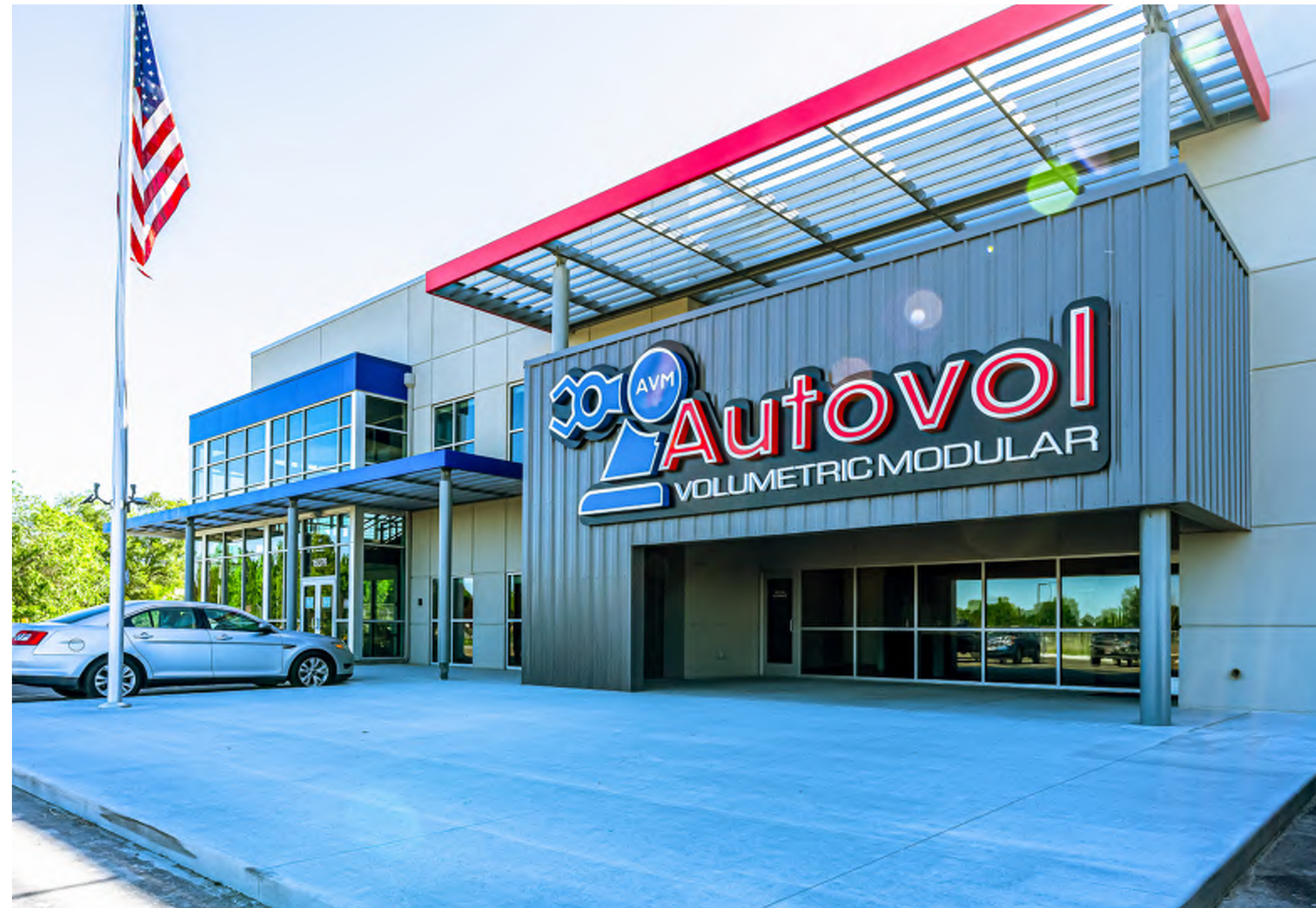
Autovol Volumetric Modular | Nampa, Idaho | ZGA Architects & Planners, Chartered
